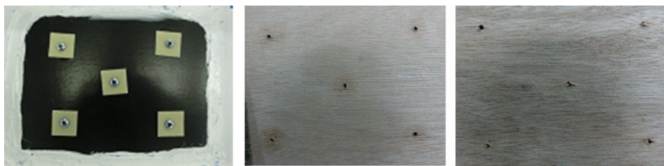
Fig.2 Appearance after AAMA screw water seal test when we placed 3040BK
